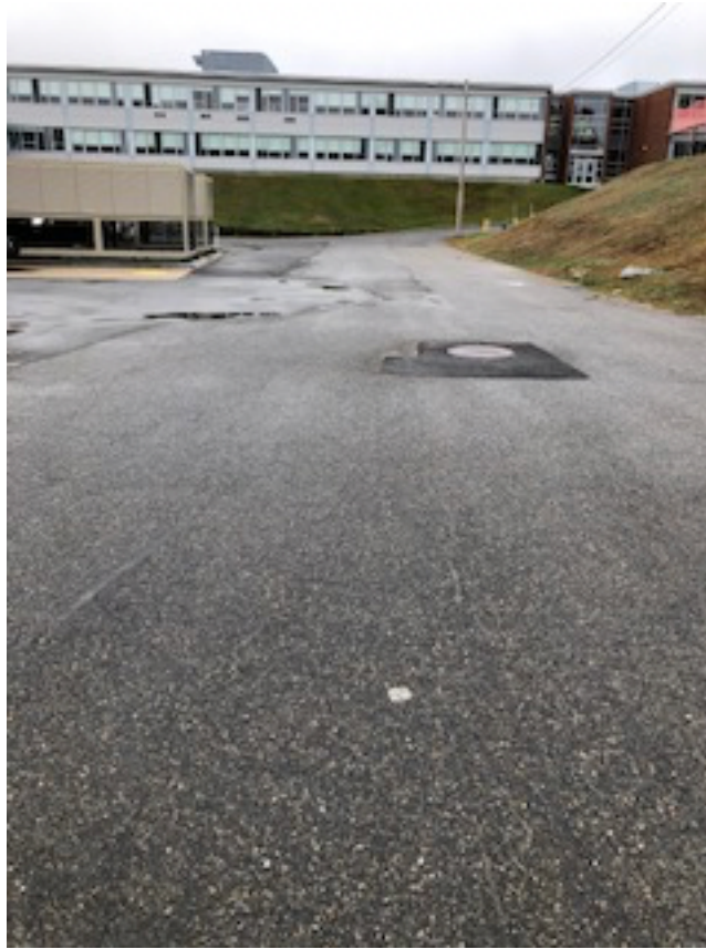
Manhole at western edge of AUL area, looking south; Athletic Field at back of school is to the right of photo
