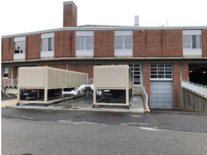
AUL area – under HVAC equipment, to left (north) of ramp
